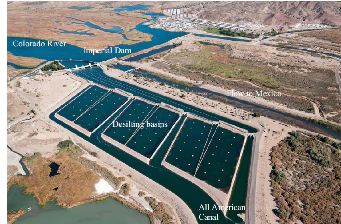
Imperial diversion dam (Courtesy of United States Bureau of Reclamation)
